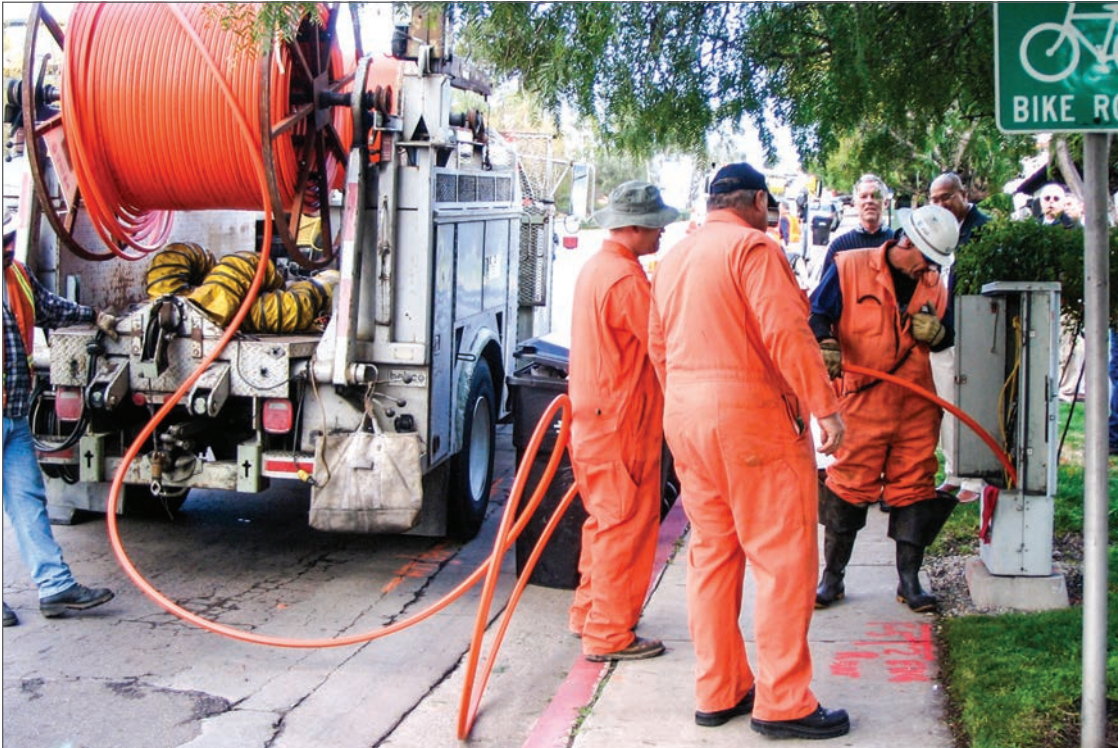
Figure 1. Microduct installation
