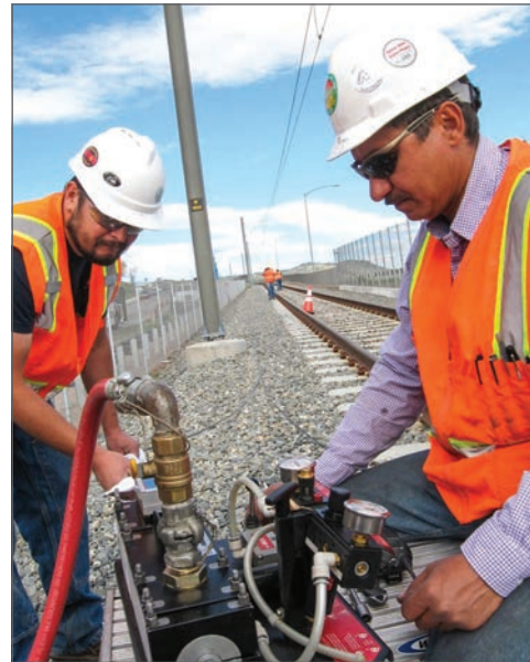
Figure 23. Micro Cable Blowing Installation
