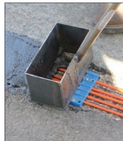
Figure 28. Microtrenching Method
