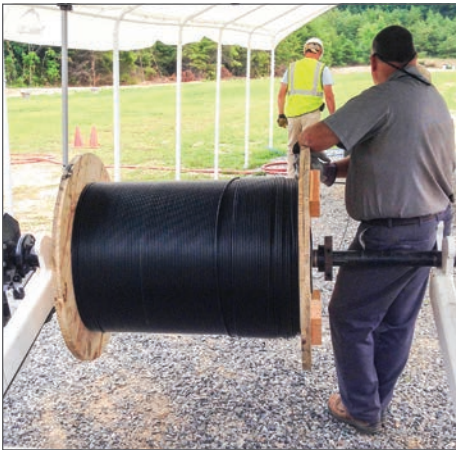
Figure 6. Payout of a 144-Fiber MiniXtend Cable
